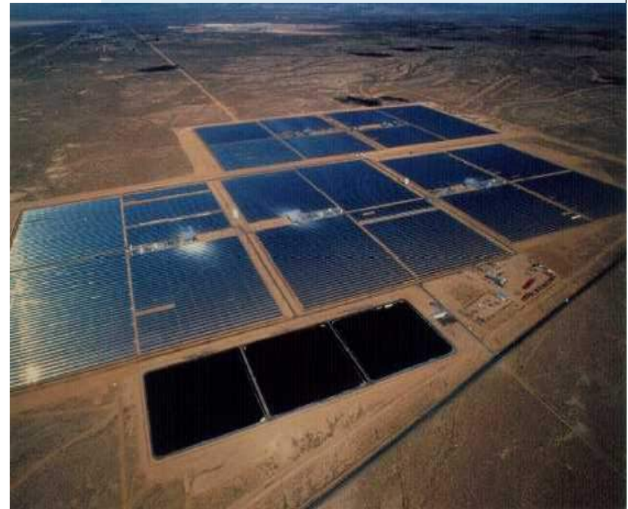
Luz / FPLE's Kramer Jct. SEGS III – VII Parabolic Trough Plants ( 5 x 30 MWe)
